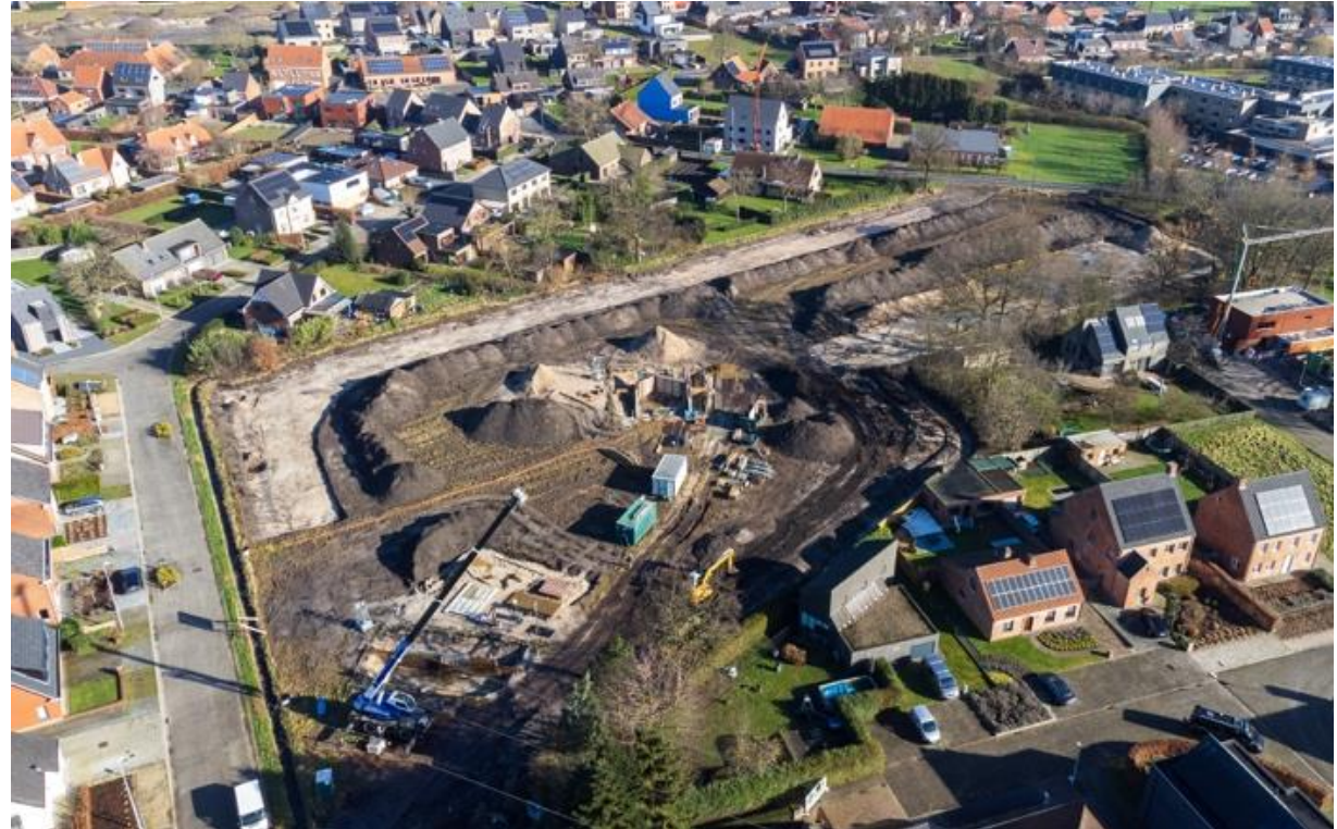
Construction of the flood retention area in Beerse, Belgium
