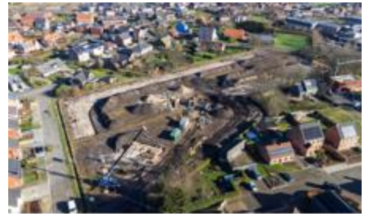
Construction of the flood retention area. Source: Province of Antwerp
